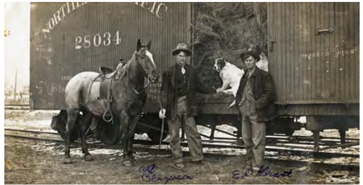
A rail car filled with wire grass ready to ship to St. Paul. The nearest rail station for the company was in Forest Lake.
