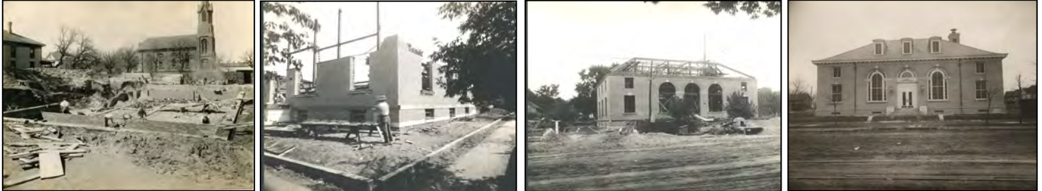
Stages of construction, 1915-1916.
