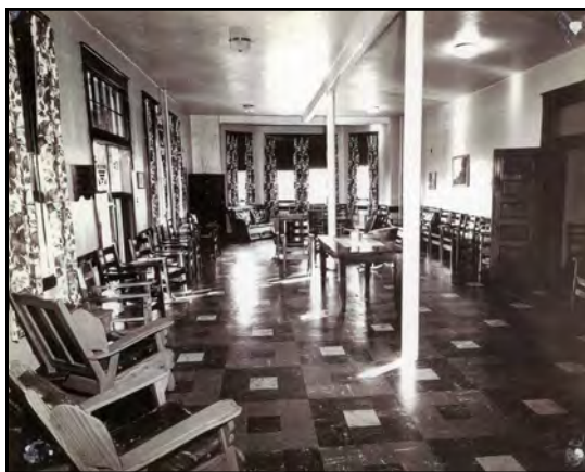
View of a common room in one of the Cottages.
